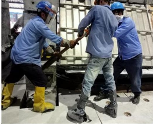
Figure 3. The previous method of tightening the shunt by hand ratchet.
